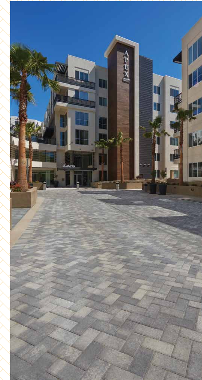
Opposite Left: Gray-Moss-Charcoal Holland installed in a herringbone pattern. Note: This stone was manufactured at 80mm due to site conditions and anticipated traffic loads. Above Left: Gray-Charcoal Holland installed in a 45° herringbone pattern. Note: This stone was manufactured at 80mm due to site conditions and anticipated traffic loads. Above Right: Red-Brown Holland installed in a herringbone pattern.
