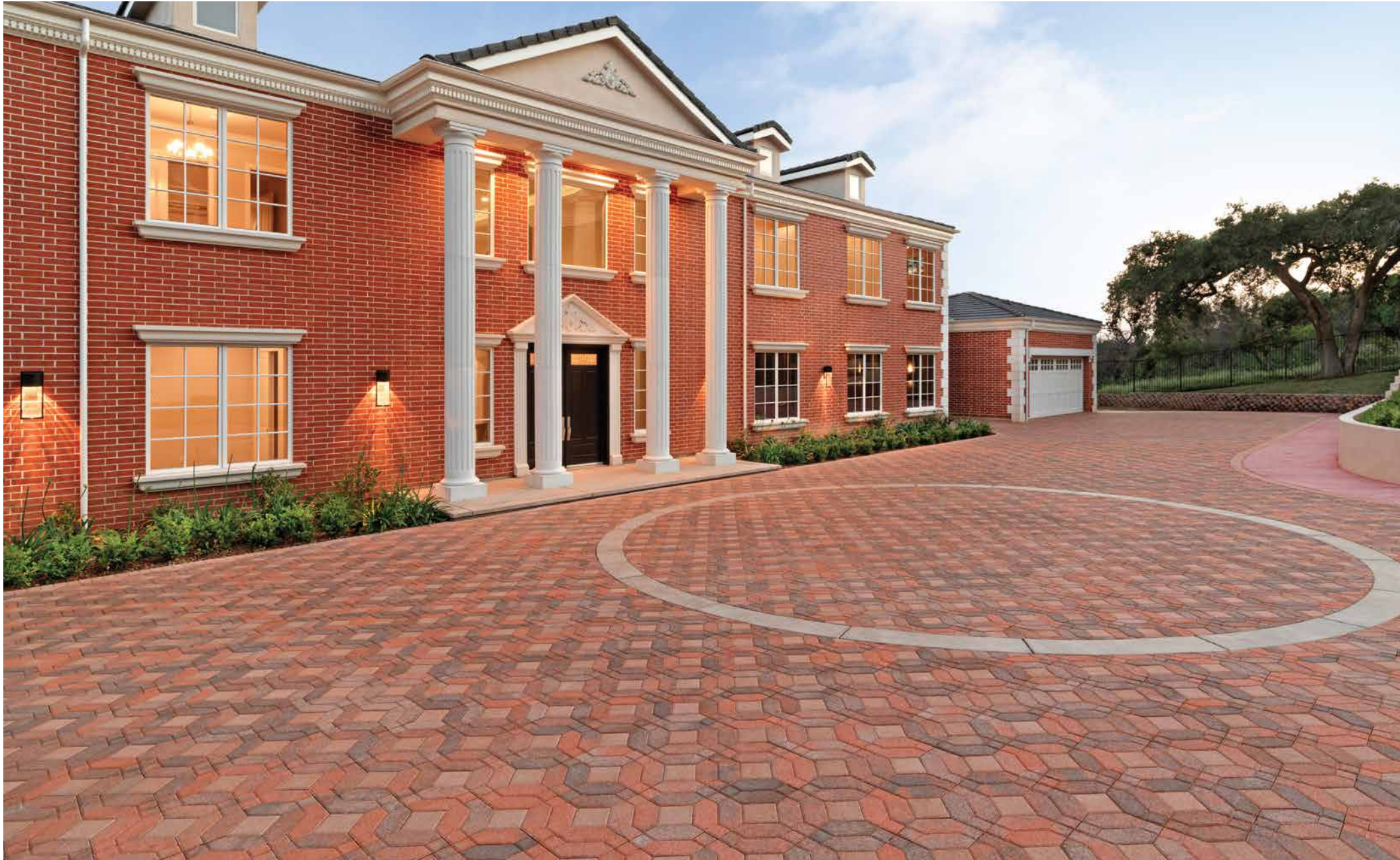
Above: Cream-TerraCotta-Brown Symetry and solid Cream 6x6 installed in a Venetian parquet pattern. Border is solid Cream Holland. Right: Cream-TerraCotta-Brown Symetry and Cream 6x6 installed in a Venetian parquet pattern.
