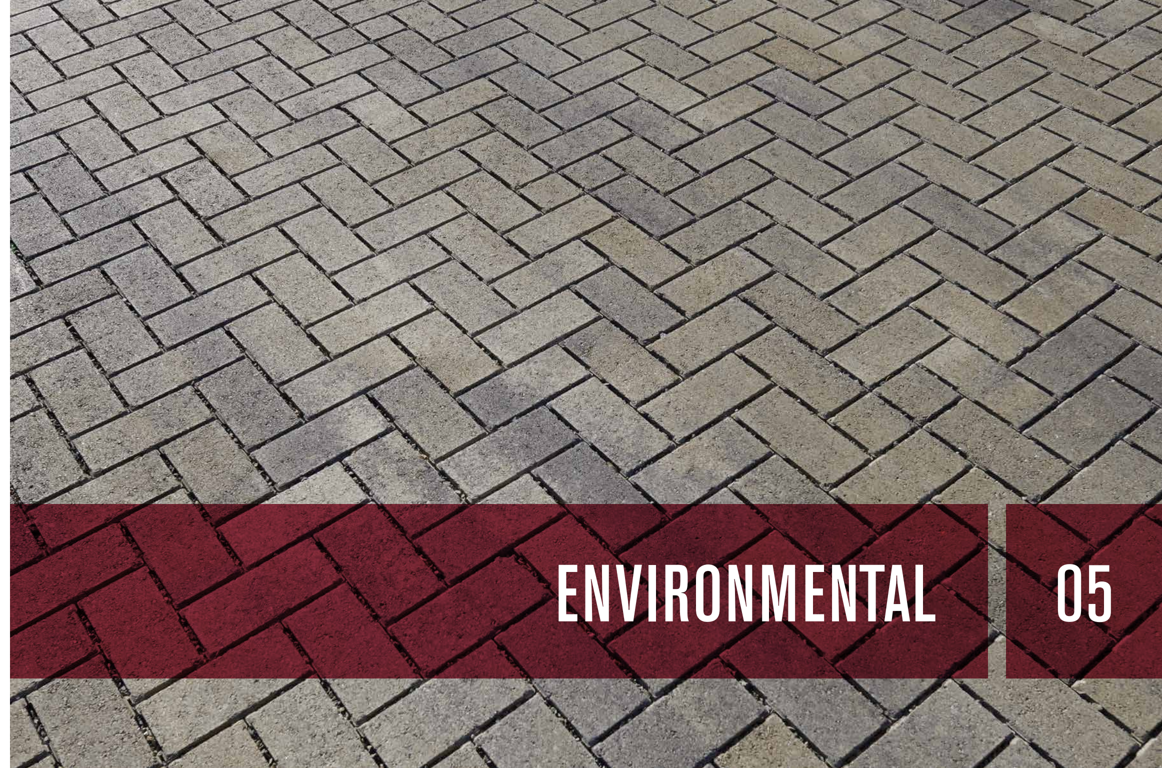
Above: Solid Mocha Permeable Holland Pavers installed in a herringbone pattern. The border-banding detail is solid Charcoal Permeable Holland installed in a soldier course. Right: Gray-Moss-Charcoal Permeable Holland machine-laid in a herringbone pattern.
