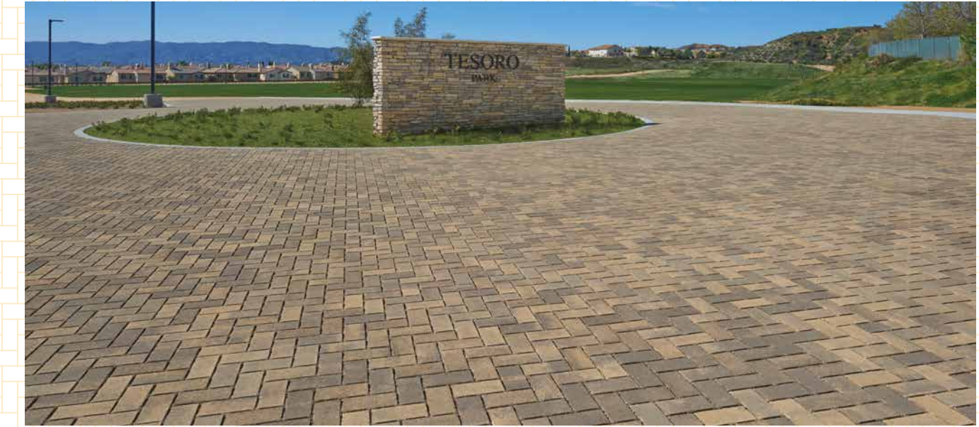
Above: Sand-Stone-Mocha Permeable Holland installed in a herringbone pattern.
