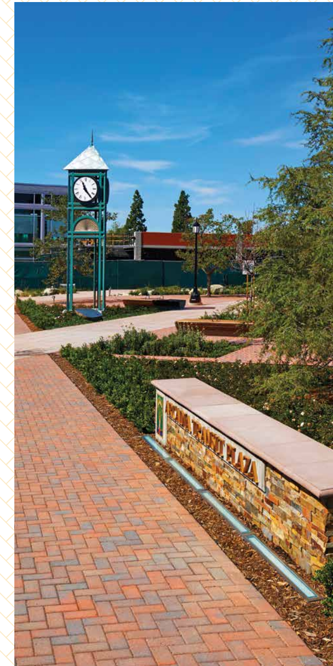
Opposite Left: Gray-Moss-Charcoal Holland installed in a herringbone pattern. Note: This stone was manufactured at 80mm due to site conditions and anticipated traffic loads. Above Left: Gray-Charcoal Holland installed in a 45° herringbone pattern. Note: This stone was manufactured at 80mm due to site conditions and anticipated traffic loads. Above Right: Red-Brown Holland installed in a herringbone pattern.
