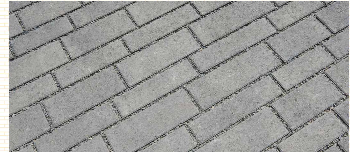
Left: Dark Gray-Pewter-Charcoal Permeable Aqualina installed in a random runner pattern. Above: Dark Gray-Pewter-Charcoal Permeable Aqualina installed in a random runner pattern. Permeable pavers are installed over open-graded base and with rock chips in the paver joints instead of sand to allow water to flow into the base underneath the pavers.
