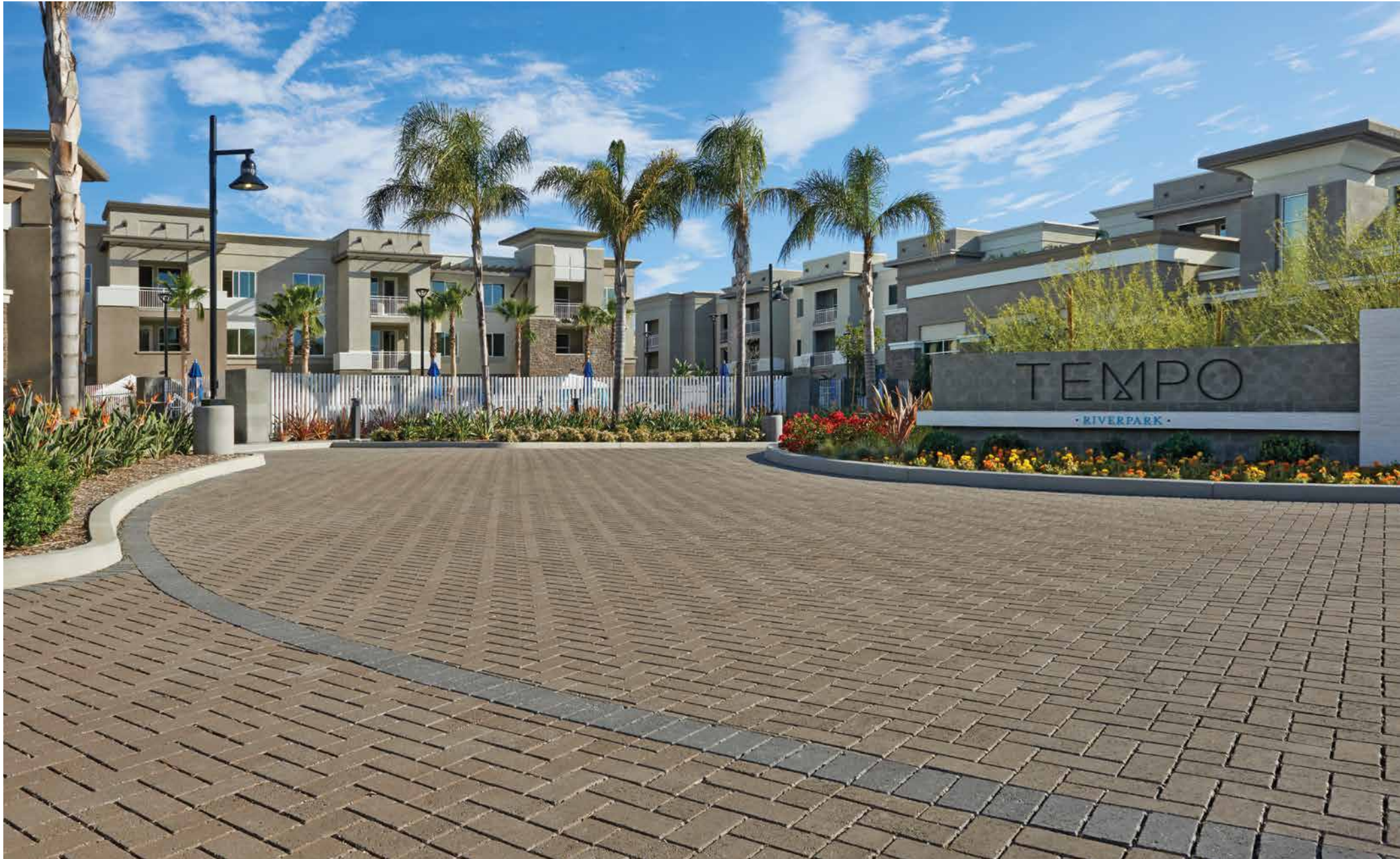
Above: Solid Mocha Permeable Holland Pavers installed in a herringbone pattern. The border-banding detail is solid Charcoal Permeable Holland installed in a soldier course. Right: Gray-Moss-Charcoal Permeable Holland machine-laid in a herringbone pattern.
