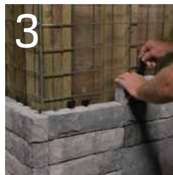
3 Attach Tandem Wall with Connector
