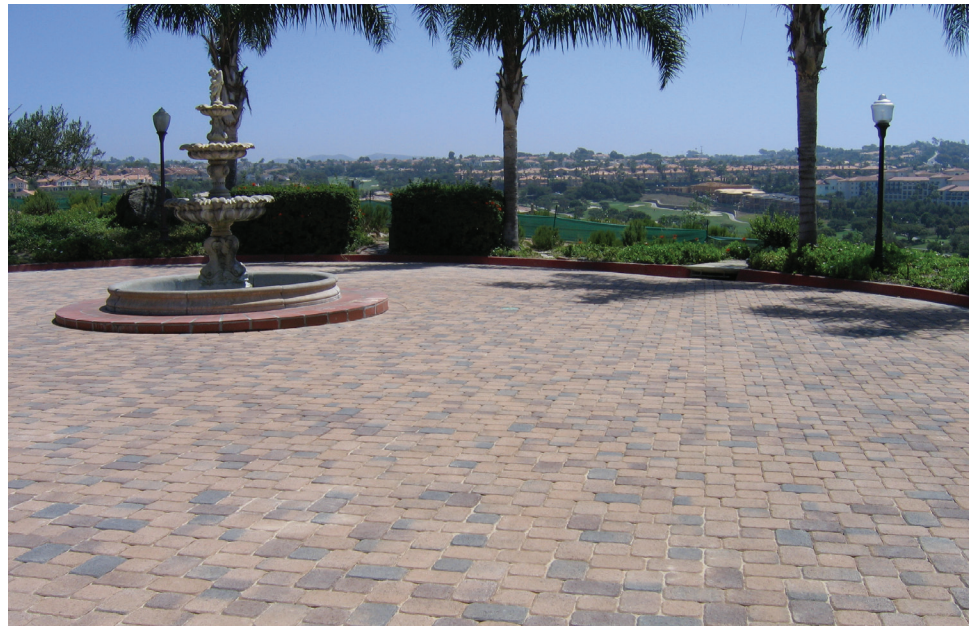
Shown: Cream-Brown and Cream-Charcoal Appian Cobble I and II installed in an “T” pattern.
