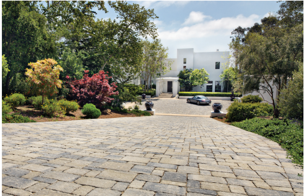
Shown: Gray-Moss-Charcoal Estate Cobble I & II (tumbled) installed in a random ashlar pattern.
